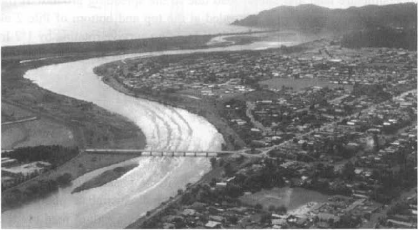
Fig. 1.11 An aerial view of the Landing Bridge.
