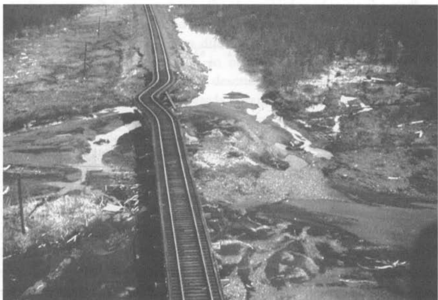
Fig. 4.2 Damage to a railway bridge during the 1964 Alaska Earthquake (USGS).
