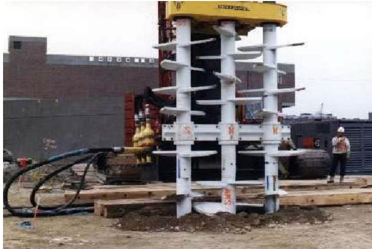
Figure 140. Photo. Typical blade-based tooling for WRS mixing. (127)
