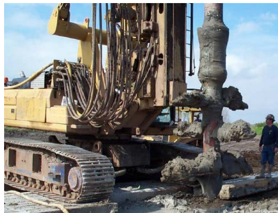
Figure 144. Photo. Typical tools used for WRE mixing.
