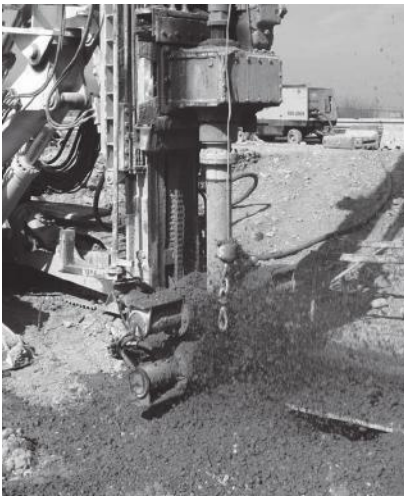
Figure 2.12 Jet grouting spoil outflow (a) and production (b).
