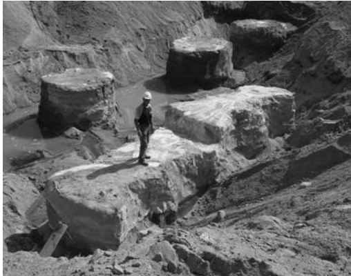
Figure 2.4 Example of candy columns. (Courtesy of Trevi.)
