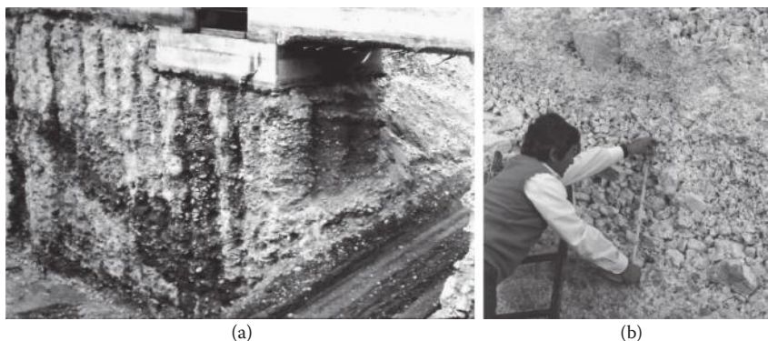
Figure 3.15 Effects of jet grouting on gravelly soils.
