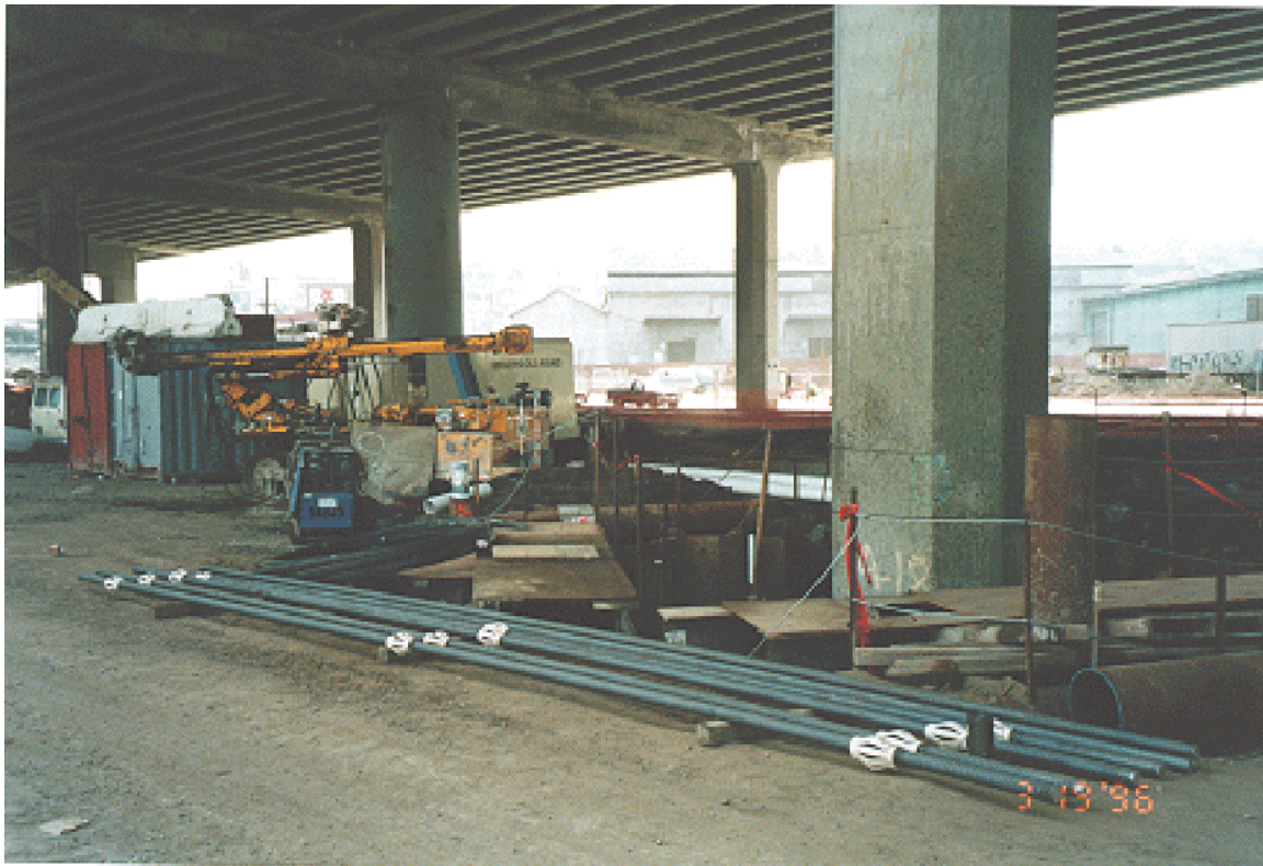
Figure 8-3. Storage of Reinforcing Steel.
