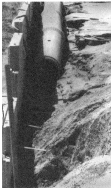
(c) Backside of wall in (b), which shows the reinforcing strips attached to the wall face units. Note the drain pipe to carry runoff from the future road surface. Recent rain has eroded soil beneath reinforcement strips at wall, which will have to be carefully replaced. Also shown are interlocking dowels and lifting devices (D rings), which weigh around 2 kips each.
