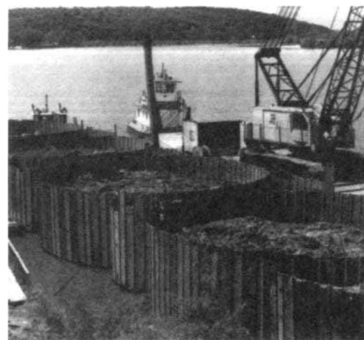
(b) Cofferdam under construction showing initial part of cell line 1-2 with cells being partially filled for stability.
