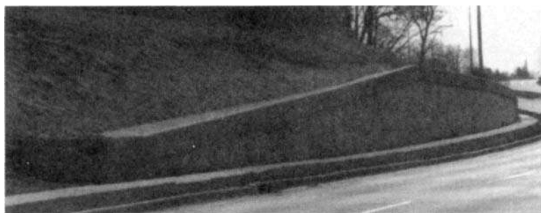
(d) A low reinforced earth wall showing a different concrete facing unit pattern (also patented). Note top cap includes a drainage depression that empties into a drop inlet barely seen at forward end.
