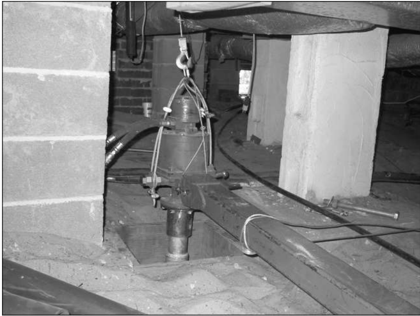
Figure 2.10 Low-headroom installation (Courtesy of Magnum Piering, Inc.)
