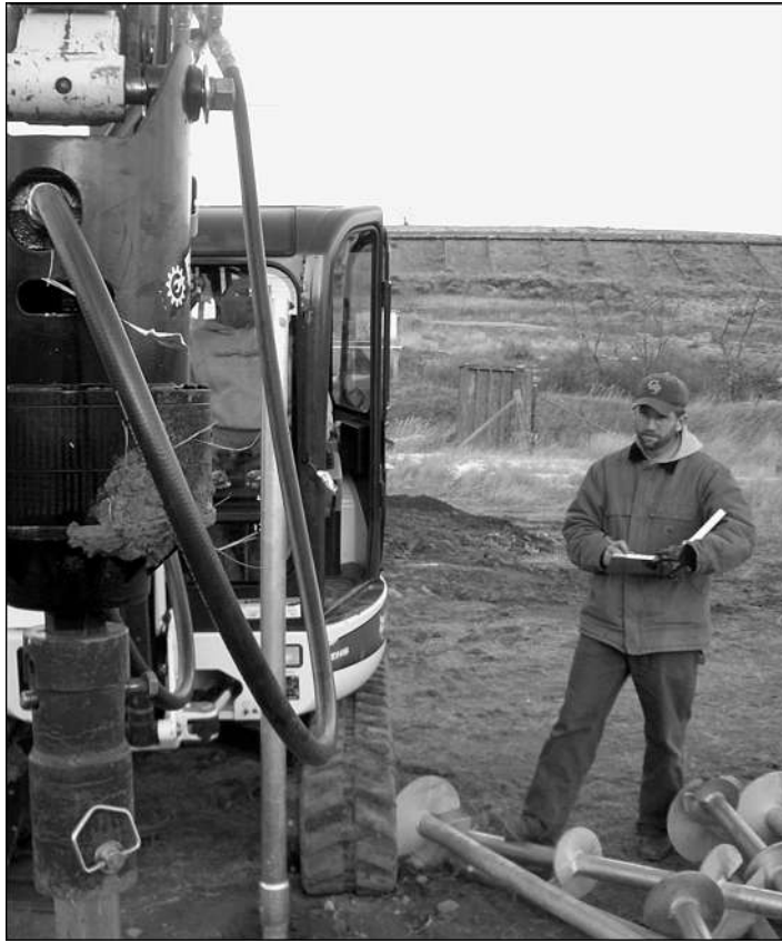
Figure 2.28 Helical pile inspection
