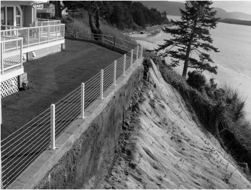
Figure 13.18 Helical soil nail reinforced slope (Courtesy of ECP)
