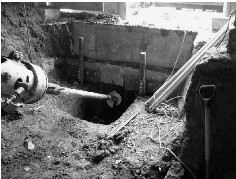
Figure 14.10 Installation of Top Row Helical Anchors (Stage 1)
