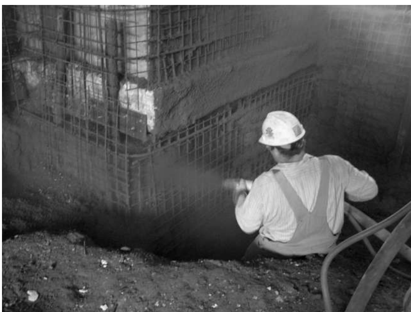
Figure 14.11 Shotcrete Application (Stage 2)
