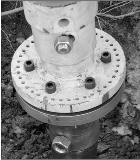
Figure 2.14 Shear pin indicator (Courtesy of Magnum Piering, Inc.)
