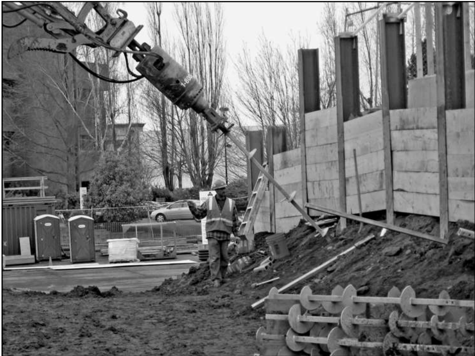
Figure 1.27 Soldier beam and lagging system with helical tie-backs (Courtesy of Earth Contact Products, Inc.)
