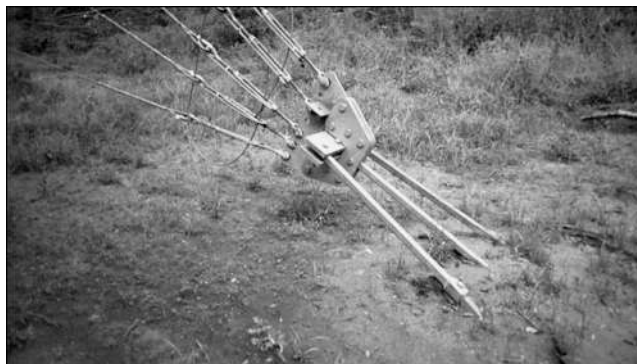
Figure 1.17 Utility guy wire anchors (Courtesy of Hubbell, Inc.)
