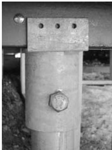
Figure 12.15 Example flitch beam cap
