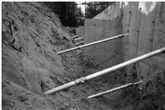
Figure 13.22 Repair of counterfort wall with helical anchors
