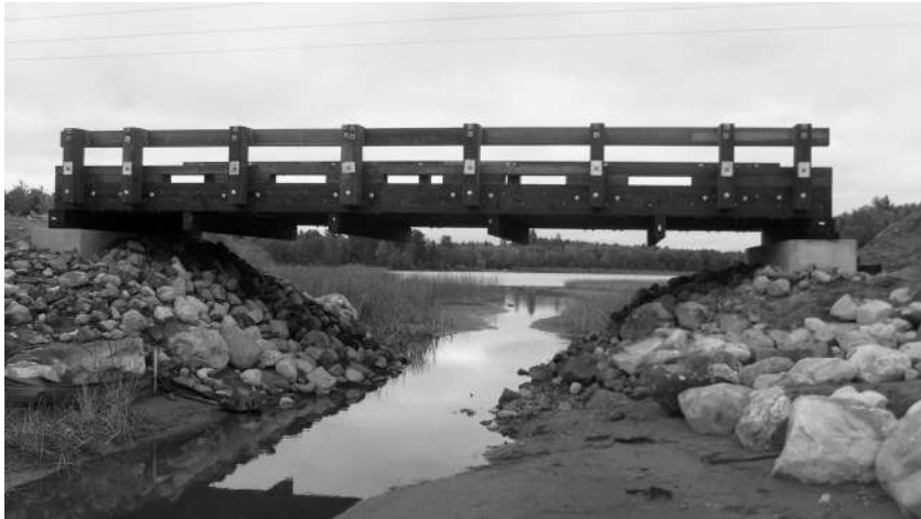
Figure 12.17 County bridge on helical foundation under construction
