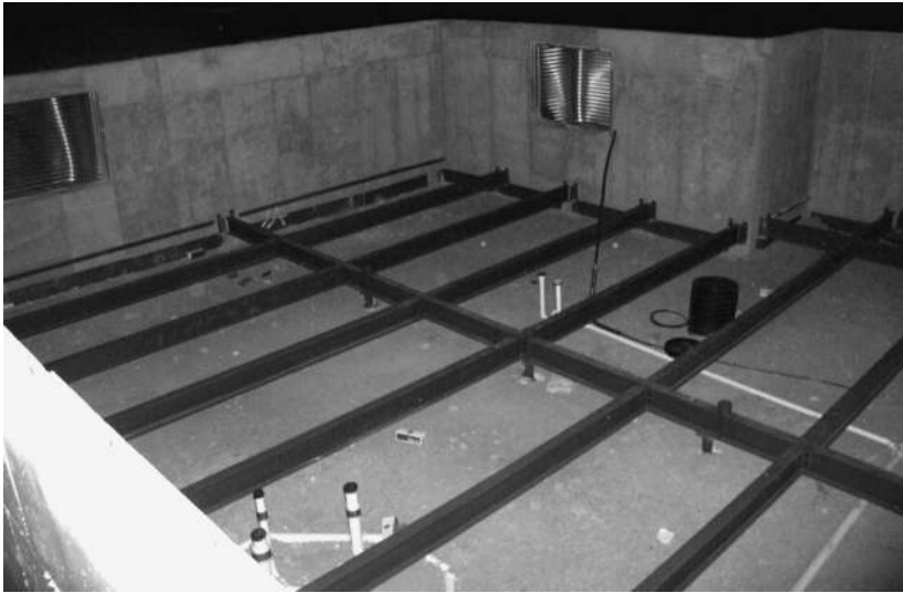
Figure 9.2 Structural floor construction on expansive soils
