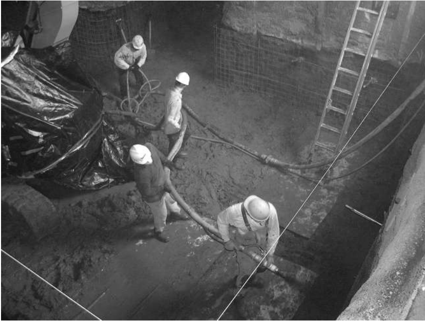
Figure 14.12 Shotcrete Application (Stage 3)
