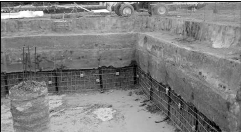
Figure 1.26 Shotcrete and helical anchor shoring system
